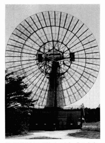
The K3NSS 25.6-meter (84-foot) parabolic reflector in the stow position. A small group from the Southern Maryland Amateur Radio Club, including the author, restored the antenna to 432-MHz moonbounce. All rf systems, including the feedlines and feed antenna, were missing. The 432-MHz system was built and installed from individual and club assets. The restoration began in the fall of 1976, and the first contact was completed with LX1DB in April, 1977.
